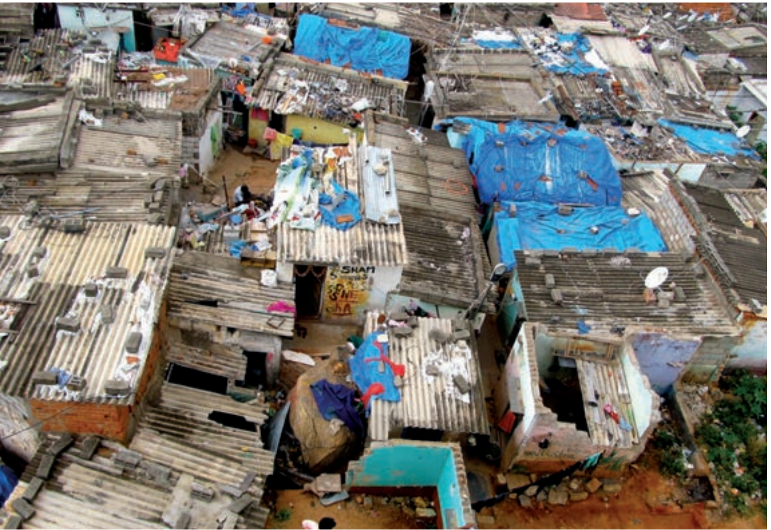
Above: The JP Nagar slums in Bangalore, India.
